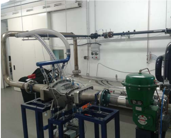
Figure 6.12: View of the Sector rig test cell
