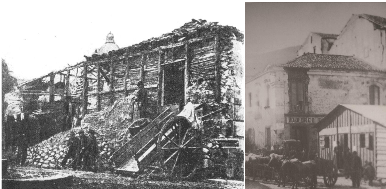
Figure 2. Seminara (Rc), 1908 earthquake; Palmi (Rc), 1908 earthquake. Overturning of the outer part of the wall, in baraccato buildings.
