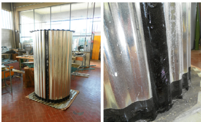
Figure 5. The prototype under construction.
