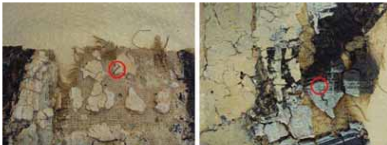
Fig. 4.8 – Metal staples on the surface of the Strip : two details
