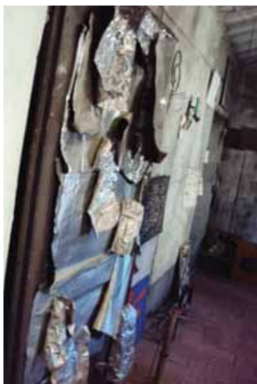
Fig. 5.2 – Aluminium foil applied on the door of the attic of Melani’s Studio-Home (image acquired on April 20, 2011)
