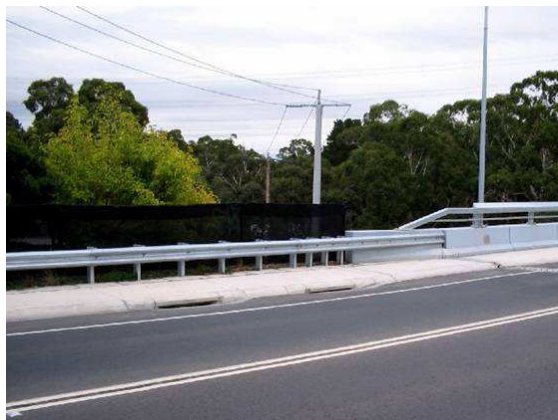
Figure 75: Transition between semi-rigid and rigid barrier [A.40]
