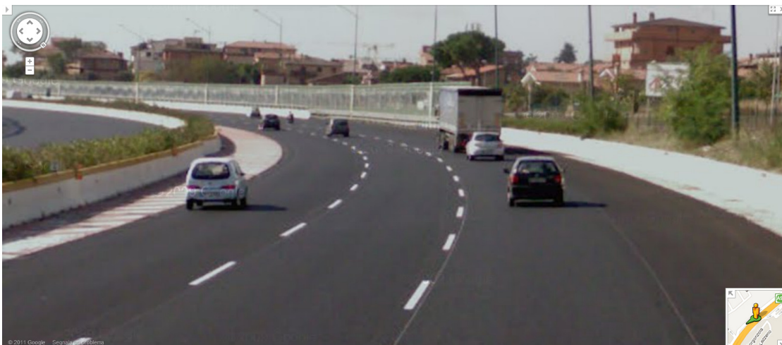
Figure 28: Raised rumble strips used in the left-hand shoulder on the Rome Beltway.
