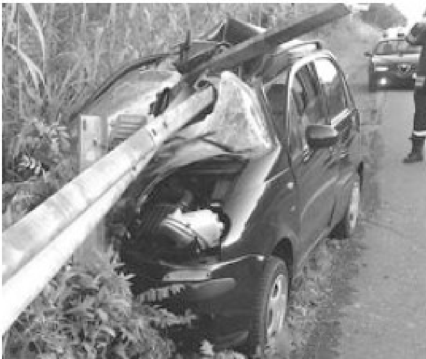
Figure 3: Head on collision with an unprotected terminal [8]
