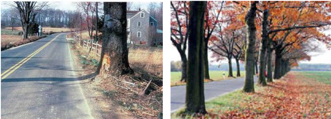
Figure 49: Examples of hazardous trees located on the roadside (Source: [A.24], [A.53])
