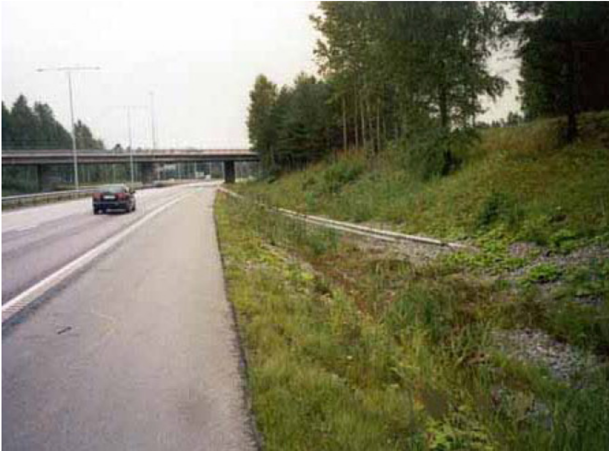
Figure 12: A buried-in-backslope terminal [1]
