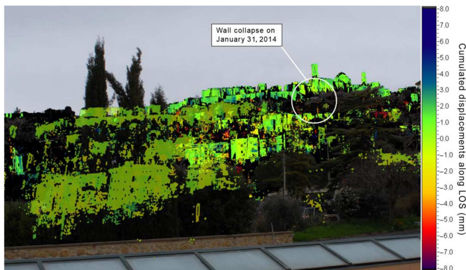
Fig. 3. 3-D radar point-cloud of cumulative LOS displacements measured by the GBInSAR from February 19, 2014 to September 16, 2014. Negative values refer to displacements toward the sensor; positive values refer to displacements away from the sensor.
