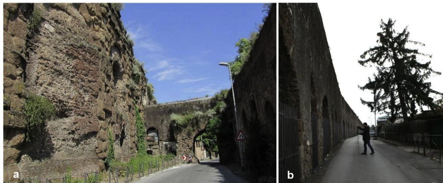
Fig. 4. Examples of a) enclosed spaces (e.g., aqueduct structures in Via del Mandrione, Rome) and b) physical obstacles (e.g., a tall tree close to the arcades of Felice Aqueduct in Vicolo dell'Acquedotto Felice, Rome) that can create practical difficulties to the collection of RTK GPS micro-topographic measurements.
