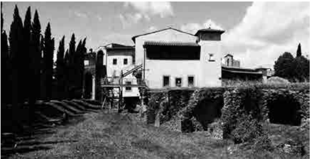
Fig. 6 – Emergency staircase. On the right side of the ambulatory south-east
