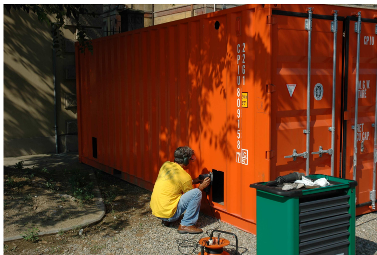
Figure 1: The container being transformed into dryer and fumigating chamber
