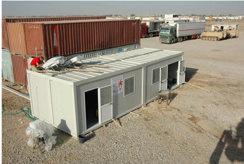
Figure 6. Date processing prefab
