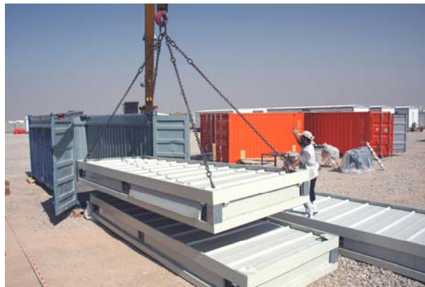
Figure 1. Modular box carrying out stage
