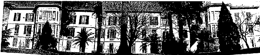
Figure 3 The Villa Ognissanti before refurbishment
