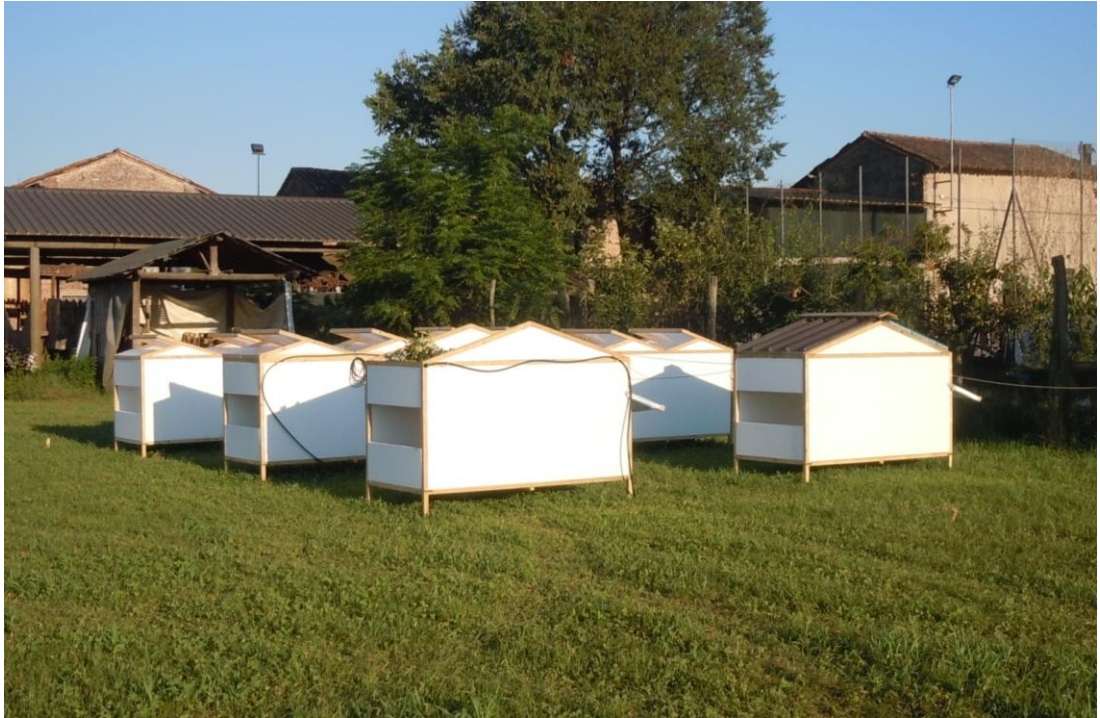
Figure 4.1. A picture of the experimental buildings taken during the tests.
