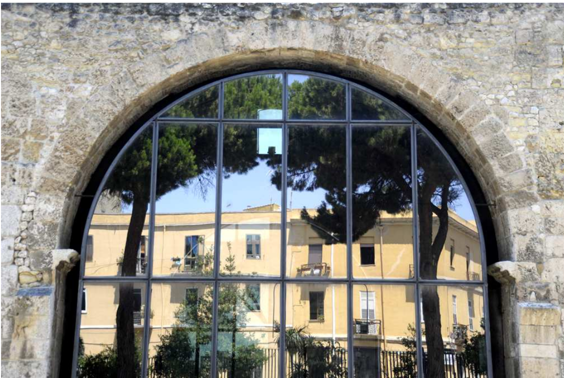
Fig. 3 – Particular of the glass walls, July 2013 (Copyright Giorgio Verdiani).
