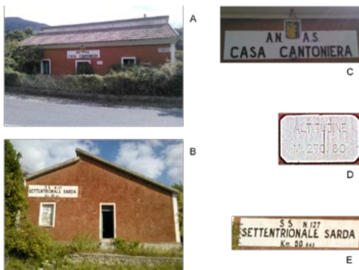
Fig. 2. An abandoned roadman's house (Northern Sardinia). A and B: two building's facades. C, D, and E: facades details. C: the typical Italian name of a roadman's house ('casa cantoniera'), decorated with the ANAS' official emblem. ANAS is the Italian acronym of 'Azienda Nazionale Autonoma delle Strade' (in English, National Autonomous Roads Corporation). D: elevation of the roadman's house above sea level (270.80 metres); letters are engraved on a plaque. E: name of the road facing the roadman's house, namely S.S. n. 127 'Settentrionale sarda': S.S. stands for 'strada statale' (in English, national road).
