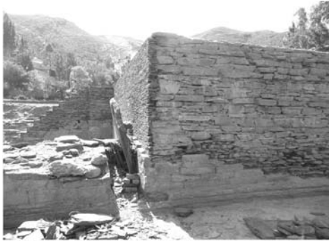
Fig. 1 Saidu Sharif (PAK) conservation work of the main Stupa
