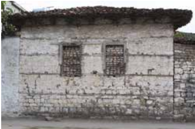
Fig. 11 Masonry building with timber hooping in Albania (photo: I. Hasa).
