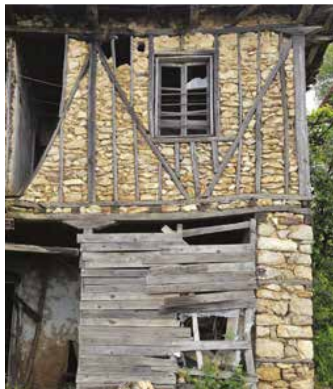
Fig. 16 House with a stone-built ground floor and a wooden frame structures with stones infill in the region of Gotse Delchev, Bulgaria (photo: S. Mecca).
