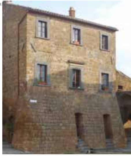
Fig. 2 Reinforcing all the ground floor at Civita di Bagnoregio, Lazio, Italy (photo: S. Onnis).
