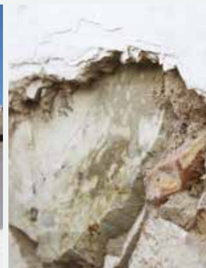
Dwellings in São Vicente e Ventosa: high thermal mass walls of stone and earth masonry (photos: I. Costa Carrapiço).
