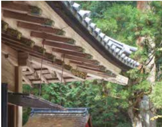
Fig. 4 The eaves in Japanese architecture prevent the sunrays from touching the house, that is simultaneously open in all fronts to catch the breeze and create a crossed ventilation inside the dwelling. Japan.
