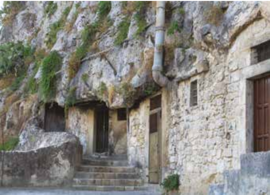
Fig.2 Underground dwellings in Scicli, Sicily, Italy.
