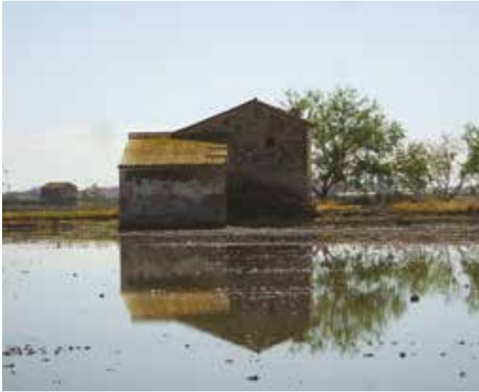
Fig. 3 House in the lagoon of Valencia, sharing two medias: earth and water, Spain (photo: F. Vegas, C. Mileto).
