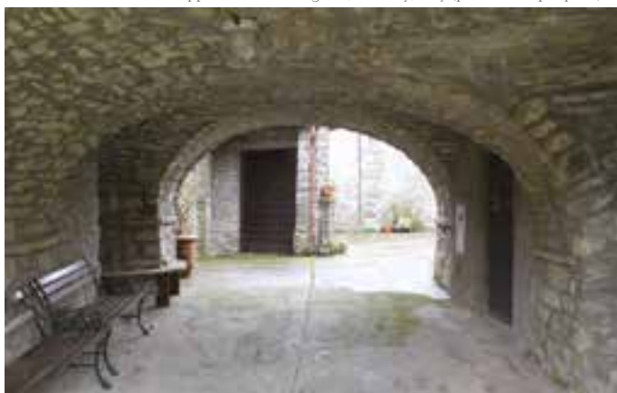
Fig. 9 Stone masonry vaults increase the mass of the building at the ground floor and create a solid connection between opposed walls. Lunigiana, Tuscany, Italy (photo: L. Dipasquale).
