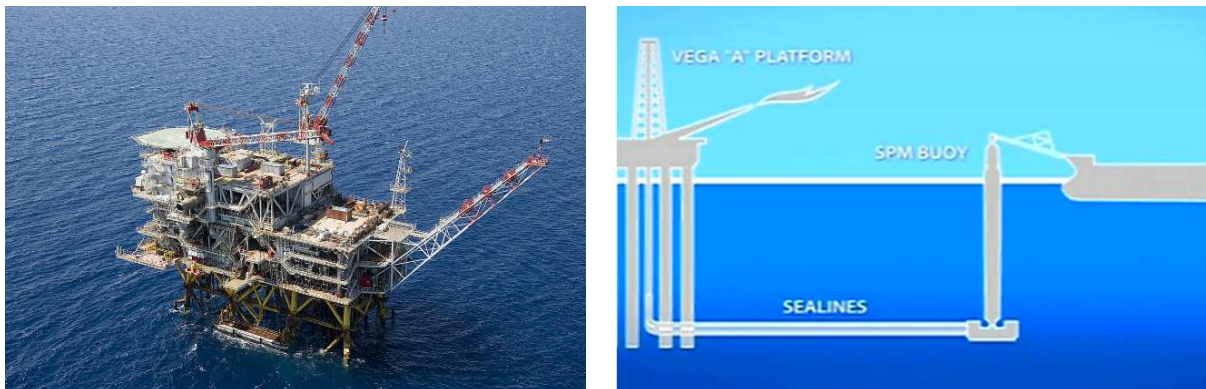
Figure 1. VEGA-A platform and FSO Leonis.
