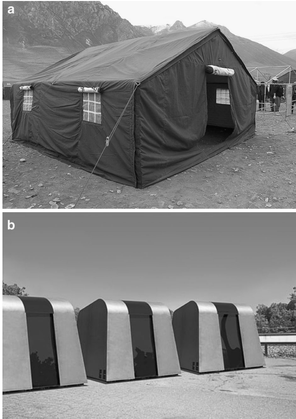
Fig. 3 Temporary shelters: a with transformable elements (source http://sichuan-quake-relief.org/ ) and b with non-transformable elements (source http://www.reactionhousingsystem.com/ )
