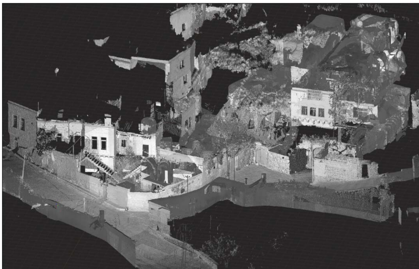
Fig. 3: Saklı and Ali Torun Kilise. Axonometric view of the complex. Point clouds.
