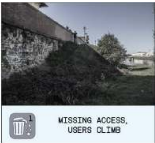
Figure 13 - Missing access, people jump or climb
