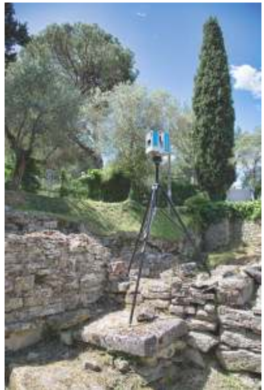
Figure 12 – 3D Laser Scanner at work in Area 1000.
