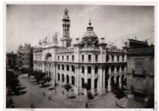
Figure 12 - Valencia 1923. Telegraphic and Postal Building (Derrey).
