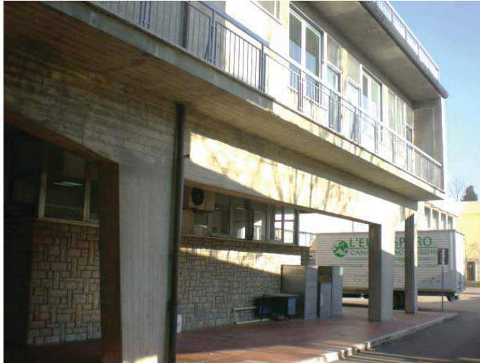
Figure 4. 4 Outdoor space of the structural unit n°15: the basement.
