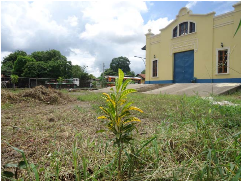
Image 2 - La Bodega de la Antigua Estación del Ferrocarril de León after the restoration carried out in self-building from the district.
