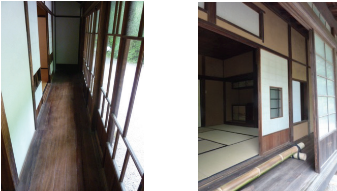
Image 3 and 4: Engawa – shoji and glass screens closed (left), and both screens open (right). © 2014 Courtesy of the author
