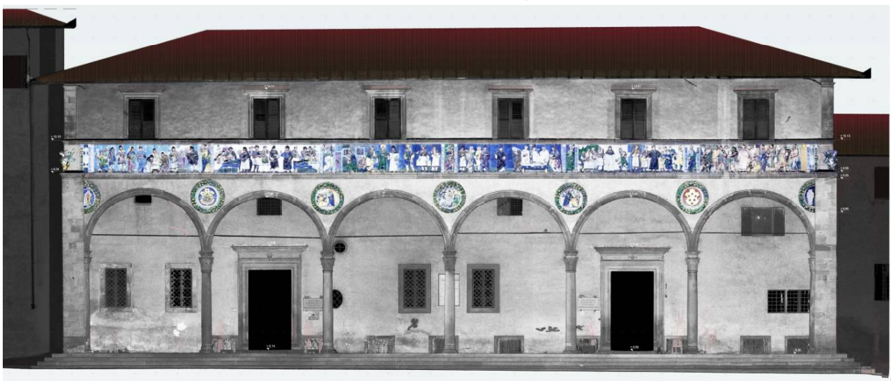
Figure 1. The main façade of the Ospedale del Ceppo, with the earthenware frieze
