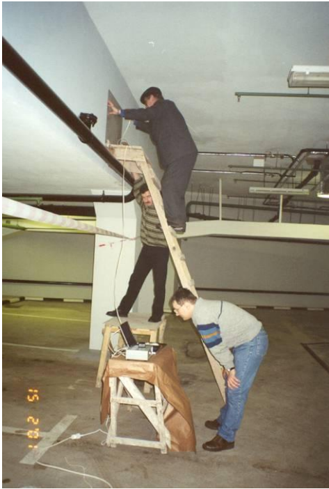
Fig. 22. Surveying of a ceiling bench in an underground garage.
