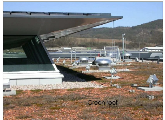
Green Roof and atrium roof [7]
