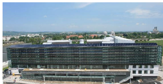
Figure 3.26: Example of PV in the façade, Energy Base, Vienna (AU) [22]
