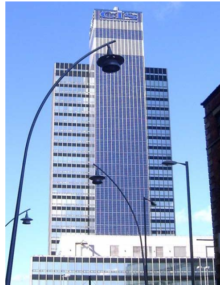
Figure 5.85: Example of building with PV on the vertical façade, CIS Tower [10]
