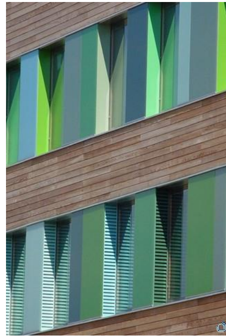
Figure 3.12: Grill for night cooling, Federal Environmental Agency, [15]
