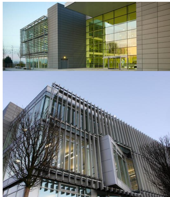
Figure 2.24: Example of office building with passive solar heating strategies, the “hub”, Atkins’ office, Bristol (UK) [16, 17]
