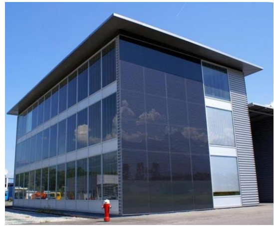
Figure 2.39: Example of cold façade, Buhler Electricité Office, designer: Kurmann & Cretton SA, Monthey (CH), 2008-2011 - Renovation, Energy production of PV on South-façade = 6000 kWh/a [32]
