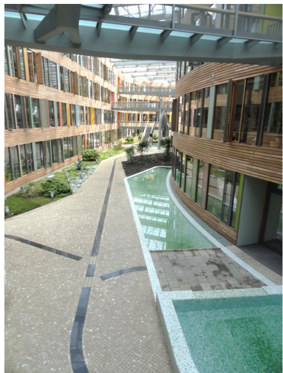
Figure 2.30: Example of evaporative cooling in office building (atrium), Federal Environmental Agency, Dessau (DE), Chapter 3 example n.2
