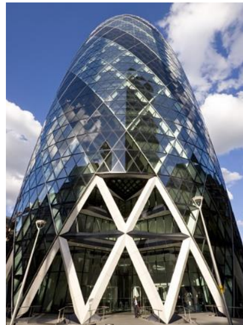
Figure 3.7: Example of high-rise building with circle geometry, Mary axe, designer: Foster and Partners, London (UK), 2004
