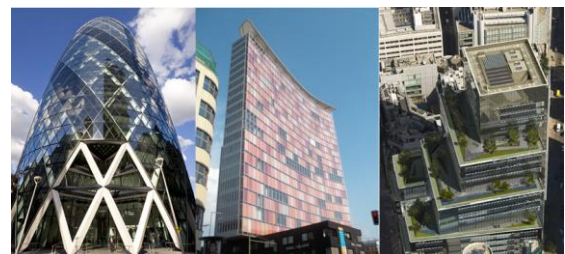
Figure 1.11: Examples of high-rise office buildings
