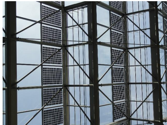
Figure 3.24: PV modules integrated into the roof of the atrium, Federal Environmental Agency
