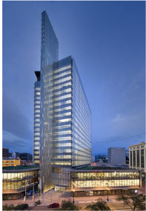
Figure 2.29: Example of solar chimney in office building, Hydro Place, Designer: Kuwabara Payne McKenna Blumberg Architects, Manitoba (CA) [23]
