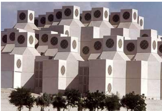
Figure 2.28: Example of wind towers, University of Qatar (QA) [22]
