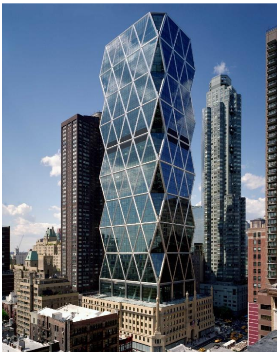
Figure 3.2: The Hearst Tower, New York City (USA), 2006. The tower, designed by Norman Foster and by WSP Cantor Seinuk (structure), is a 46-storey tall (182m) with 80000m 2 of office space. The building received the 2006 “Emporis Skyscraper Award” as best skyscraper in the world completed that year. It is first green high-rise office LEED Gold in the city and the main sustainable aspects are: - minimizing overheating with the envelope that has high performance low-emission glass with roller blinds to reduce glare and the building is also naturally overshadowed by the surrounding; - diagrid structure uses 20% less steel and it is built using 85% of recycled steel; etc. [5]
