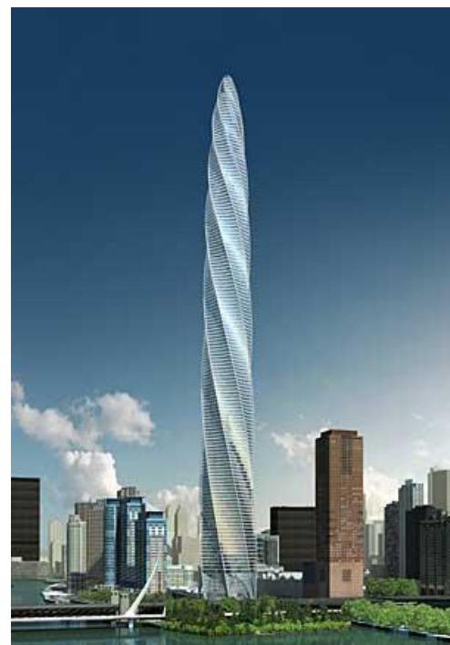
Figure 3.8: Example of twisted building, Chicago Spire, designer: Calatrava, Chicago (IL) [12]
