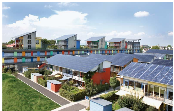
Figure 2.35: Solar settlement, Freiburg (DE), 2004 [1]
