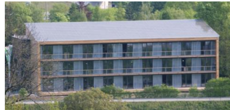
Figure 5.78: Marché International Support Office, Kempththal (CH) [9]
