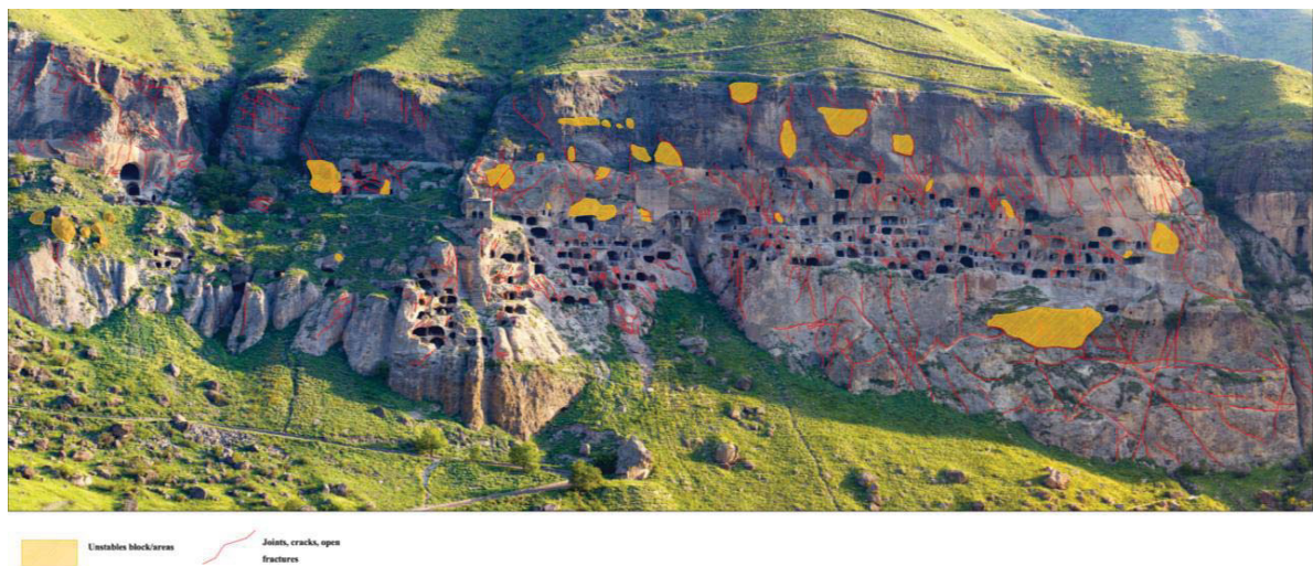
Fig. 7. Joints, cracks and unstable blocks in Vardzia cliff.
