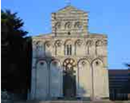
Fig. 2- San Pietro di Sorres Romanesque Church (Borutta, central-north Sardinia). The photos show the facade and the abside constructed in bichromy mainly with ashlars of local limestone and subordinately basic volcanic rocks (basalts).
