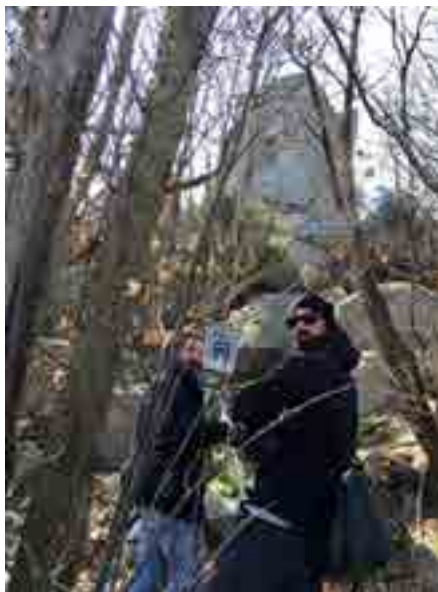
Fig. 2- Survey of the Tower of St. Giovanni in Campo nell'Elba , View of the operations (Mirco Pucci, 2016).
