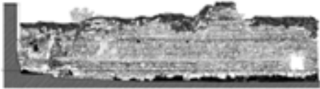
Fig. 3- View of A-A Facade (K. Bagbanci, Yilmaz, 2010).
