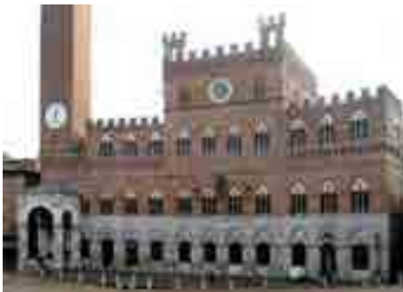
Fig. 2- Main façade of Siena Town Hall (Tuscany).
