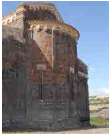
Fig. 4- San Pietro di Bulzi (north Sardinia) with abside constructed mainly with ashlars of local Oligo-Miocenic volcanic rocks and subordinately limestone for decorative ashlars.
