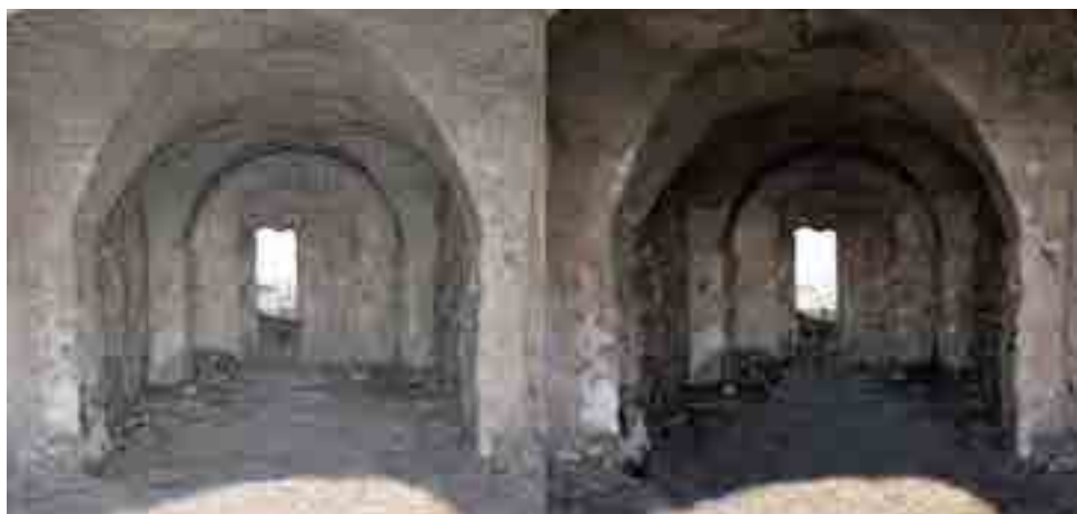
Fig. 7- The 3D model of the San Leonardo Church. Left: simple mesh – Right: the full textured mesh.
