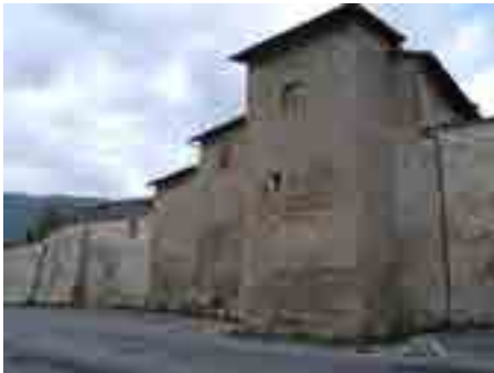
Fig. 7- Norcia, south-west side walls.
