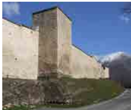
Fig. 4— Estern side walls. Remains of Roman structure.
