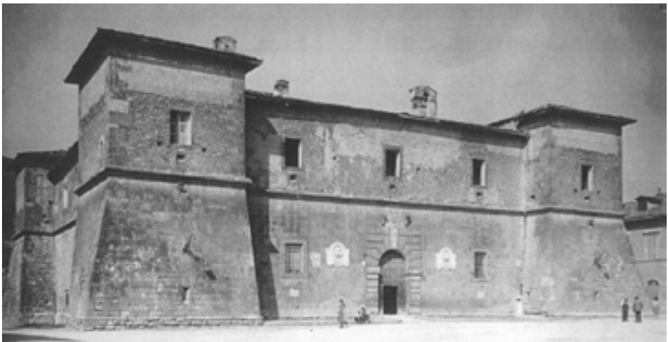
Fig. 9- Norcia, La Castellina fortress, main facade early twentieth century ( D'Avino, 2009).
