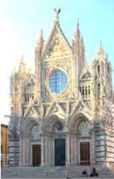
Fig. 1- Main façade of the Siena Cathedral (Tuscany).
