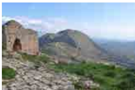
Fig. 3- View of the tower and the castle of Corinth in the background.
