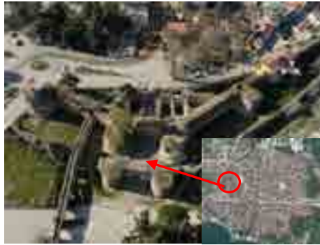
Fig. 1- Location of the Lefke Gate and Nearby Walls (Bursa Metropolitan Municipality Archive, Google Earth, 2011).
