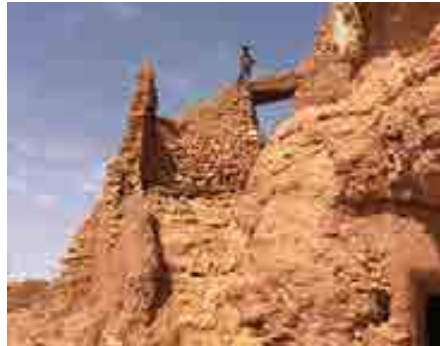
Fig.13- Palm log bridge in Taguelzi (Illili Mahrour, 2015).
