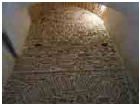
Fig. 4- Reinforcement arches (Author, 2015).
