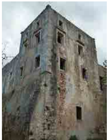
Fig.3- Tower-house in Mikro Metochi (Emma Maglio, 2014).
