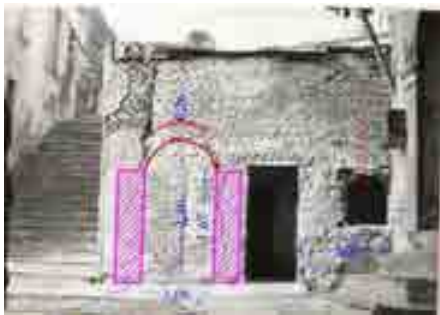
Fig. 7- Traces of a bathroom adjoining the cold room (Nacereddine Makhloufi, 2014).
