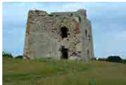
Fig. 2- The tower from the lake side.
