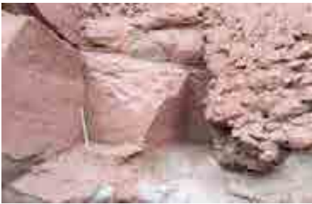
Fig.11- Aghem Taouersit. Tooling traces at foot perimeter wall (Illili Mahrour, 2015).
