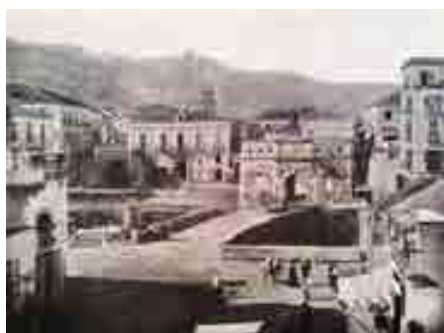
Fig. 6- De Luca, The castle square , 1860 ca. The image shows the square after the demolition of the castle (Filangieri, 1929).
