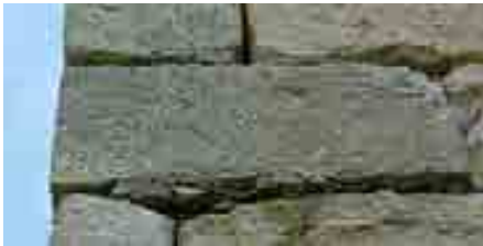
Fig. 8- Toothed chisel traces on stone blocks.
