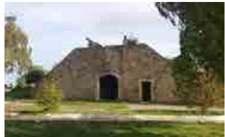
Fig. 1- view on the battery of the Caroubiers before its demolition, Annaba ( http://annaba-patrimoine.com ).
