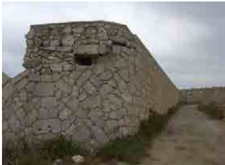
Fig. 10- PD2: all perimeter defences have at least one MG opening and one observation opening.
