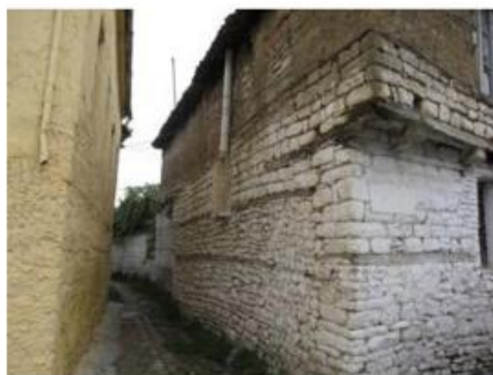
Figure 11. Stone masonry reinforced by horizontal wooden timber ties (credits: L. Rovero).
