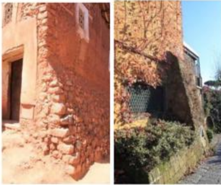
Figure 3. Buttress of random rubble masonry in Asni, Morocco, and buttress made of ashlar masonry in Naples, Italy (credits: L. Dipasquale).
