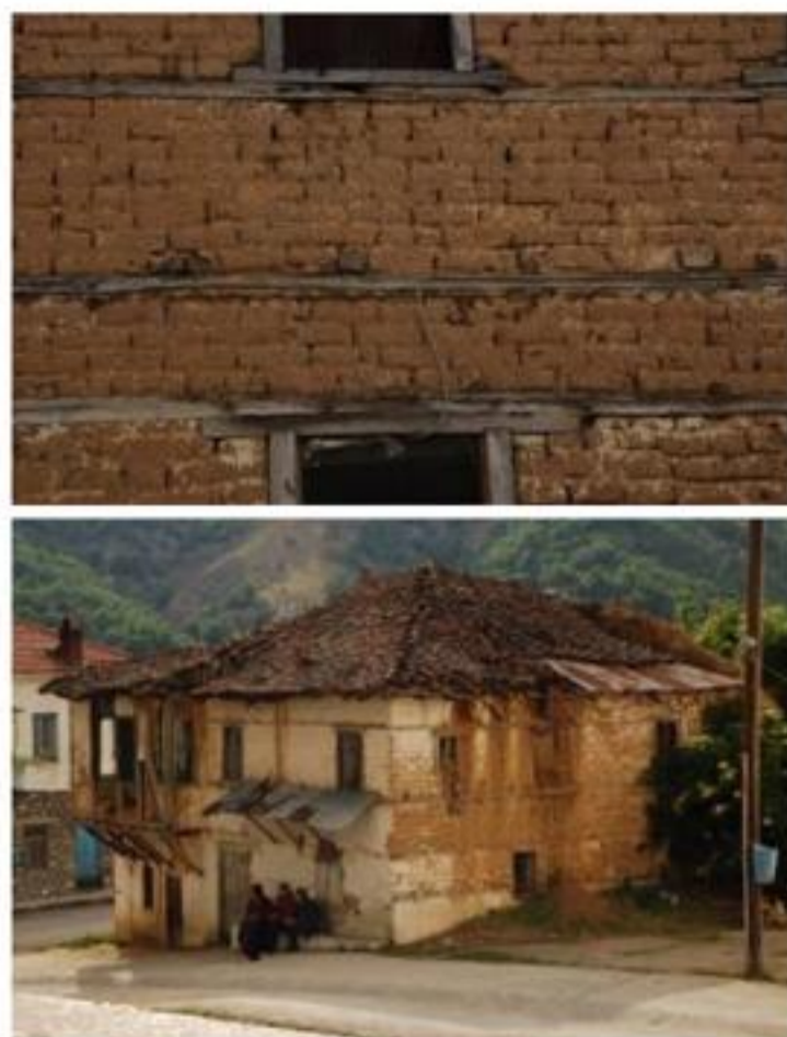
Figure 10. Two storeys adobe building with timber ties in Kastaneri, Greece (credits: S. Mecca).
