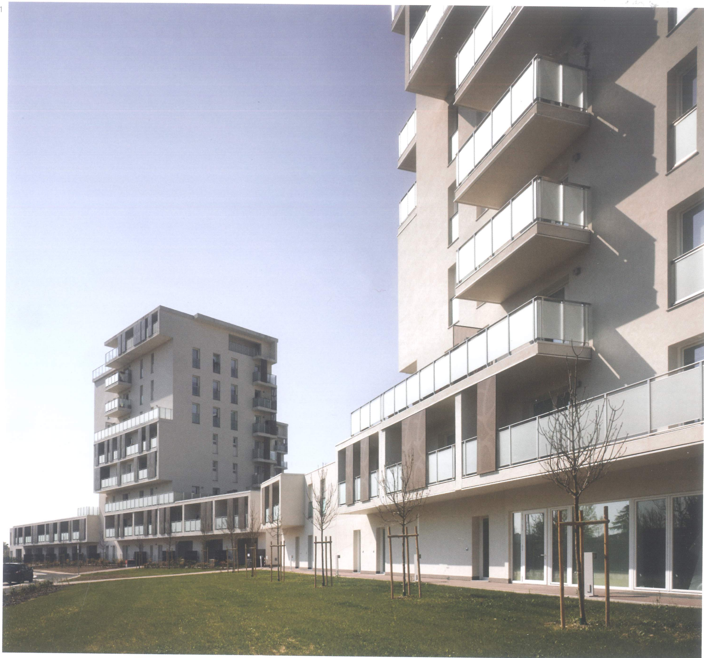
1 Vista da via Domokos View from via Domokos
