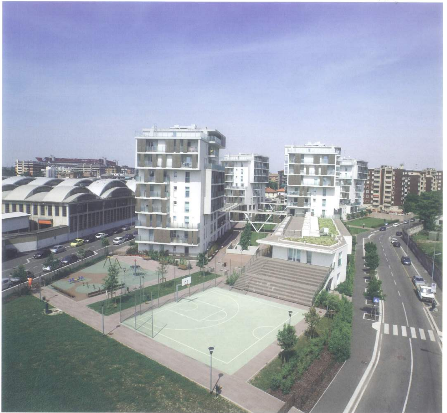
6 Vista della corte interna View of the interior courtyard
