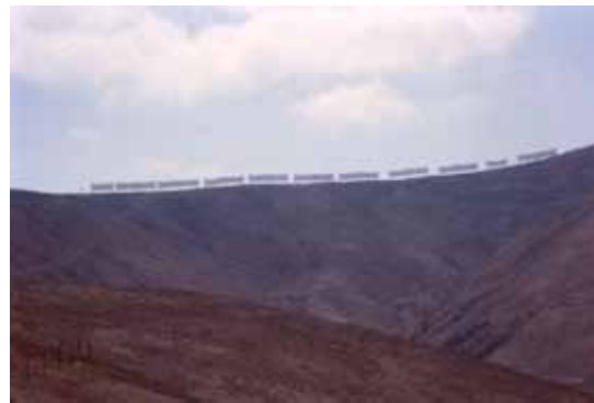
Figure 15 Fog collectors in Lomas de Meija (Source: Bresci 1997)
