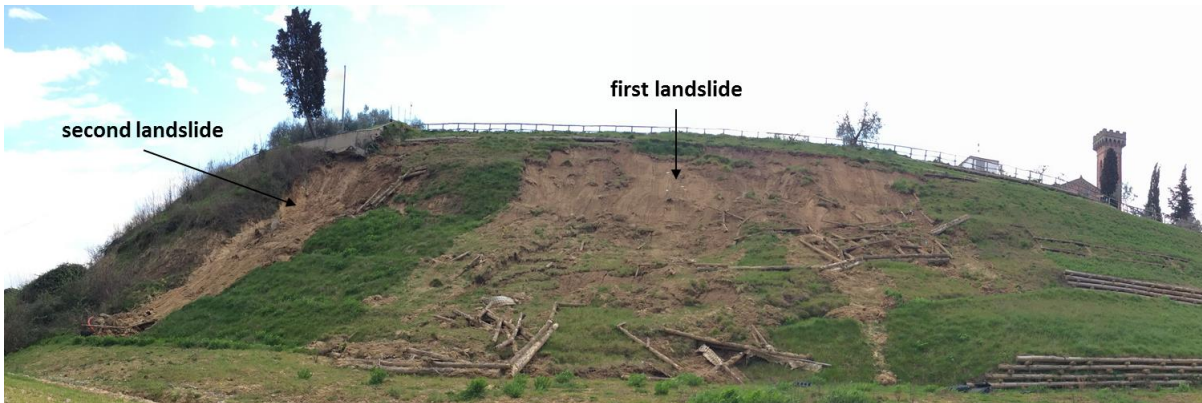
Figure 45. Northern slope of Ricasoli village with indicated the two landslides occurred in 1 st March (on the right) and 9 th March 2016 (on the left), respectively.
