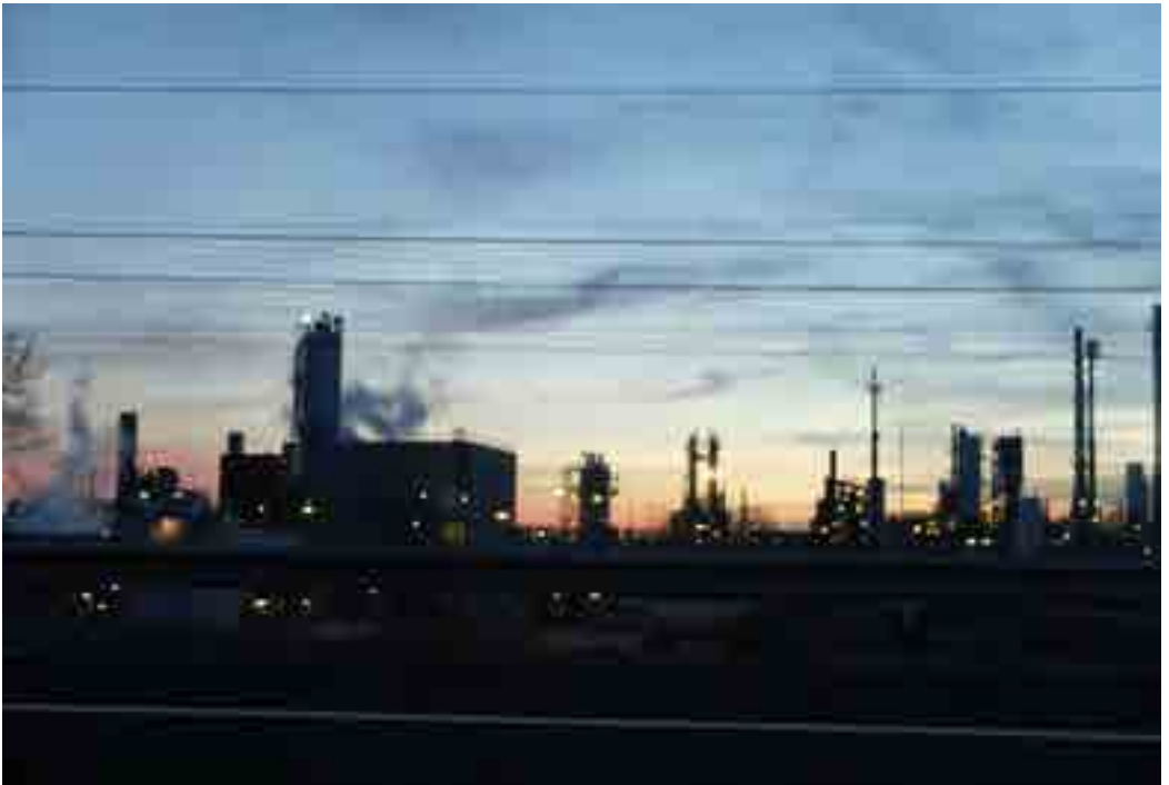
Fig.2 - View of the port of Rotterdam where the structures and productive activities of the port prove to be incompatible with the city
