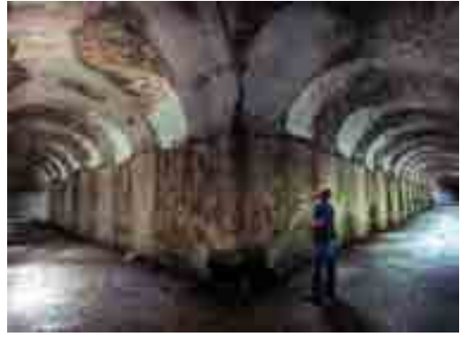
Fig. 6 - View of the cryptoporticus around the building called "Peschiera" in the Hadrian's Villa, Tivoli (G. Verdiani, G. Corsaro 2010).
