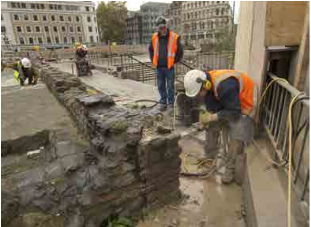
Fig 5 - Dismantling the 1962 reconstruction using diamond tipped chainsaws
