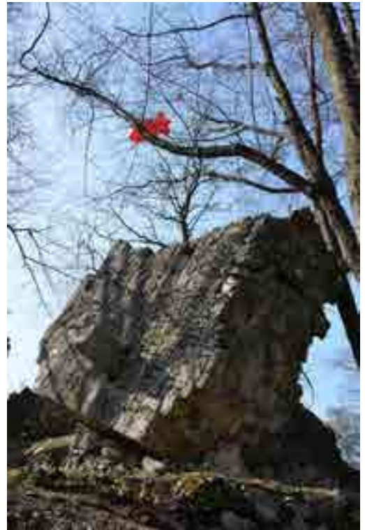
Fig. 11 - One of the fragments of the Northern Tower in Montecastrese during the aerial survey (G. Verdiani).
