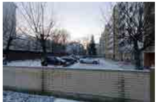
Fig. 8 – The costs of excavations on this backyard turned out to be an obstacle for making the area more attractive and comfortable. The car park underground remains undone and the area will be reserved for cars instead of recreation of the residents.
