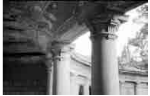
Fig. 30 - Detail of the columns of the porch in the Corallo Baths (G. Verdiani, 2012).
