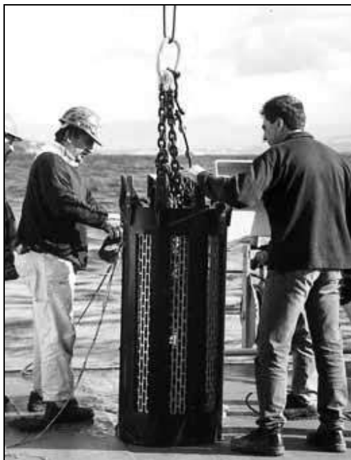
Figure 2.10 -The dredging system.
