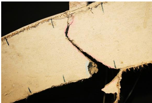
Figure 4.21 – Hinge at the extrados of strengthened arch
