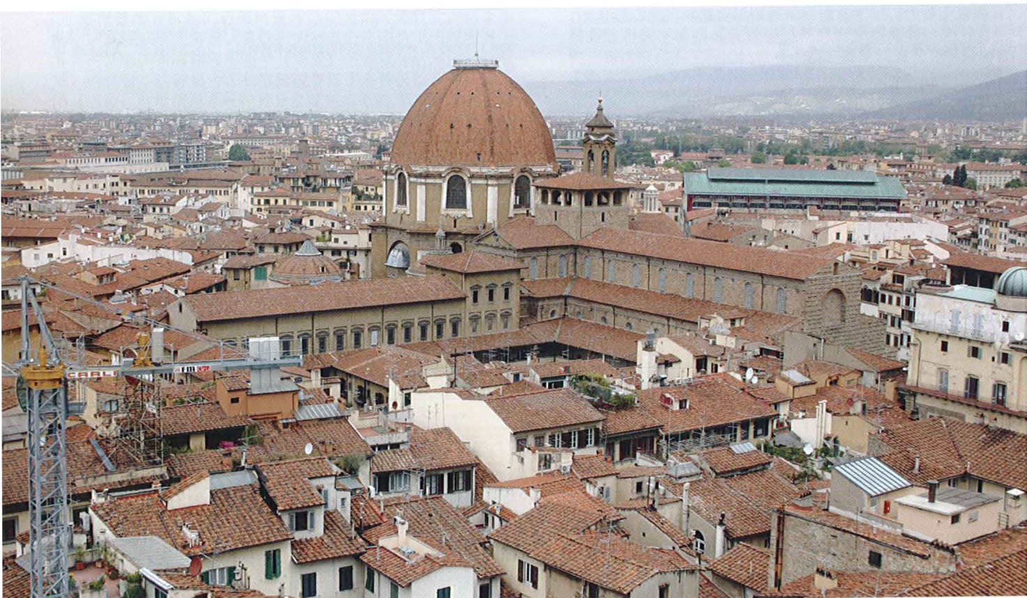
Fig. 1. View of St. Laurence complex in Florence
