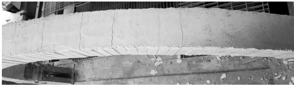
Figure 5. Superficial cracks on lime matrix, where hinge 2 formed on the un-strengthened arch.
