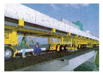
Other smart solutions like temporary 'bridges' are used to roof over maintenance work, thus relieving congestion, reducing the need for diversions and creating safe conditions for the workers'<sup>34</sup>.
