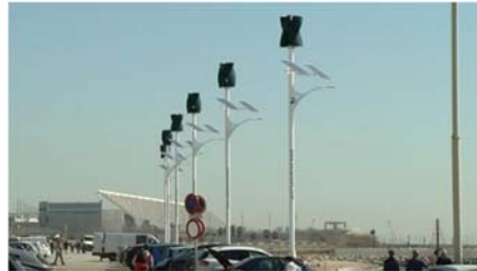
Figure 1. Street light powered by solar panels and SSWT in Barcelona northern beach. Source: Reuters link here (retrieved: 10.3.2016)
