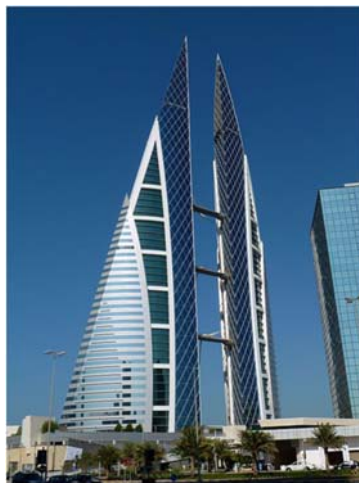
Figure 1: Urban Wind Turbines: Bahrain World Trade Center Towers. ( https://commons.wikimedia.org/wiki/File:Bahrain_World_Trade_Center.jpg?uselang=&equal:nl )
