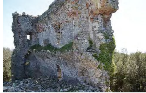
Fig. 6- Fortress of Giove - The interior façade, with the remains of the vaulted ceiling (A. Mancuso 2017)
