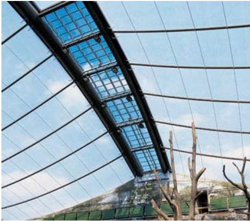
Fig.10 Fully transparent, and open in the central part to maximize natural ventilation of the site
