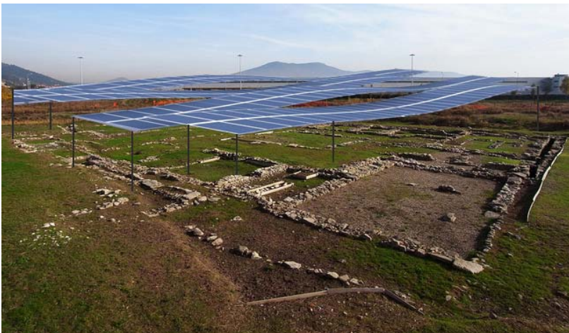
Fig. 16 One of the analysed solution for the Gongienti archaeological site with a PV roof
