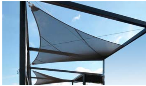
Fig. 9 This cover is realized in a stretchable water tight fabric insures an easy protection against sun and rain. The stretchable fabric
