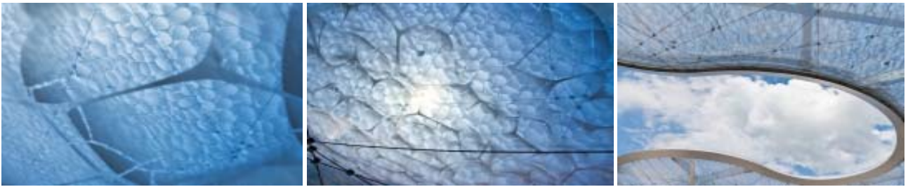
Fig. 3,4,5,6 Efte example of membrane, the air-tight cushion offers shelter while bringing light through its transparent form - photo by Niklaus Spoerri
