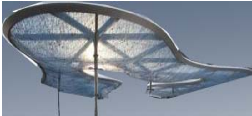
Fig. 3,4,5,6 Efte example of membrane, the air-tight cushion offers shelter while bringing light through its transparent form - photo by Niklaus Spoerri
