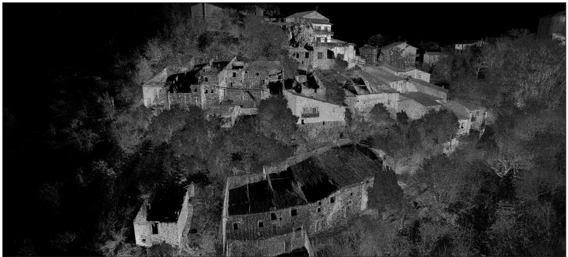
Snapshot of point clouds view of the laser scanner survey of the Acciano's center.
