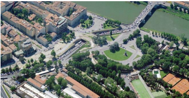
Fig. 10: The impact of contemporary infrastructures at the entrance of the Cascine Park
