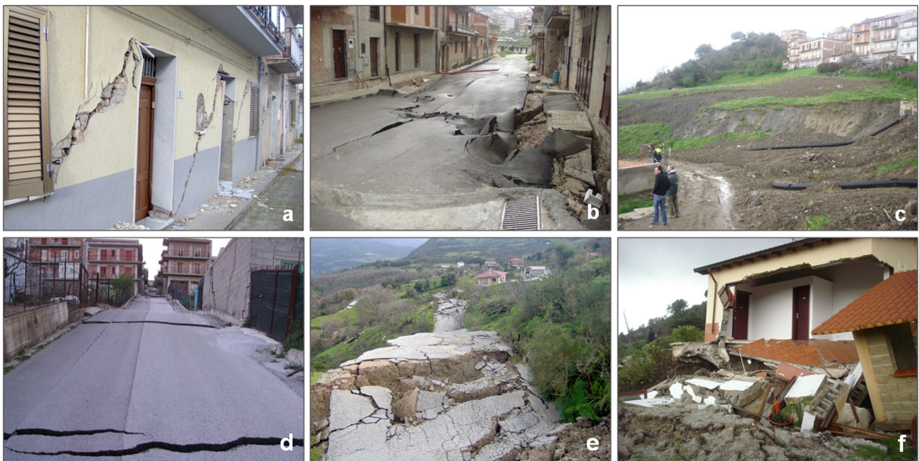
Fig. 3 Example of ground deformations and damage to buildings and structure in the 2010 landslide area. Stazzone quarter: a oriented extensional cracks on building facades and b damaged asphalt road pavement; Riana Quarter: c landslide scarps and d : traction cracks in road pavement; San Benedetto-Porcaro quarters: e country roadway complete failure and f building total collapse (see also Bianchini et al. 2015 for detailed building damage description)
