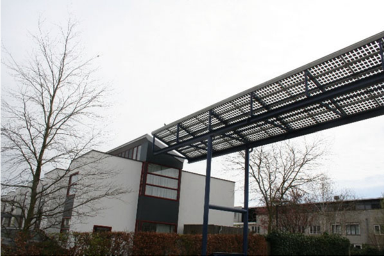
Fig. 2.6 PV integration in Amersfoort, Newland, Netherlands. Photovoltaic roof integration, Foster & Partners
