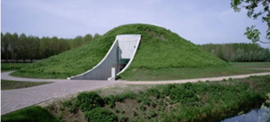
Fig. 2.2 Environmental building, Netherlands
