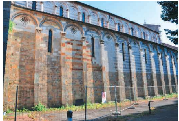
Fig. 3 – North side of the Church.
