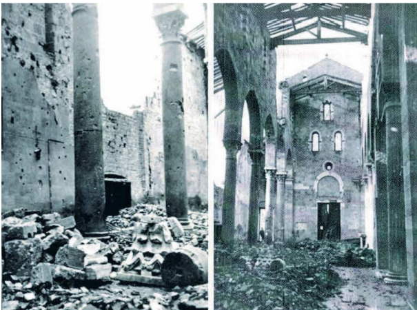
Fig. 2 – Damages due to bombing of 1943.
