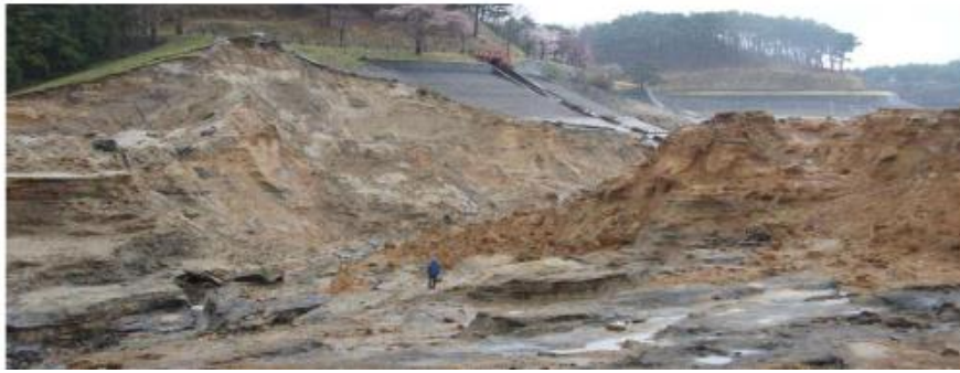
Figure 1.2 Fujinuma Dam Section after earthquake (GEER 2011, photo L.F. Harder)
