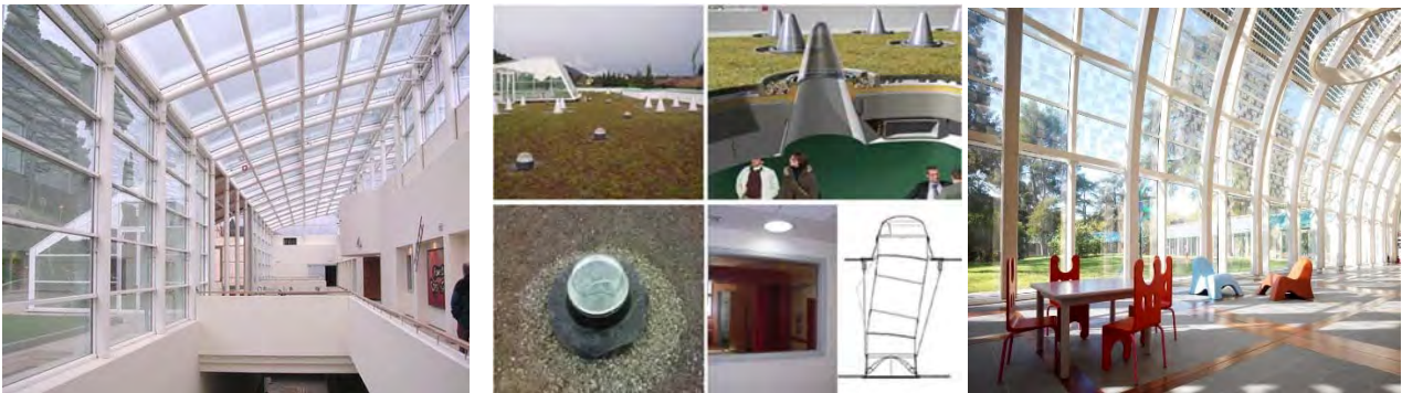
Figures 3 North corridors and greenhouse Figures 4 Solar pipes and skylights Figure 5 PV facade
